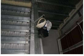
Notes: Please specify single or 3 phase motors to be used while ordering. Other shown models available. Excess water drains off from the shroud thru garden hose to drain or outside, standard water hose hook up, runs on standard water pressure. Water softener required if high mineral content is present. Rated at 5-10 gph per unit output is expected, adjustment range is 1-30 gph. Solenoid valve is \$110 vac.
