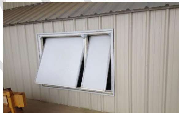
Exhaust doors in "open" position
