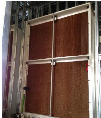
BTU stationary evaporative cooler 8' W x 12' H
