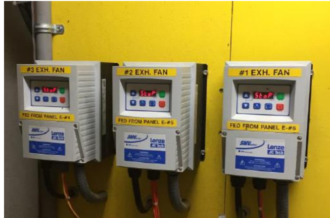
Exhaust fan VFD's (Nema 4, 2hp/1ph/230VAC 3ph)
