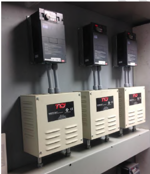
5hp VFD's and line reactors for main circulation fans
