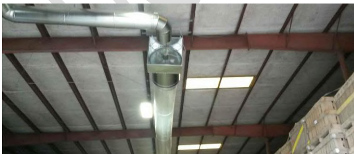
Heat distribution fan and poly tubing punched with holes for even distribution
