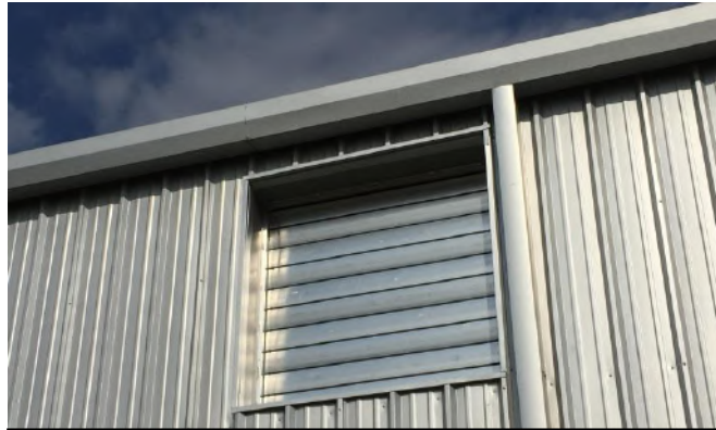
Ultra low leakage aluminum intake louvers with rubber gaskets
