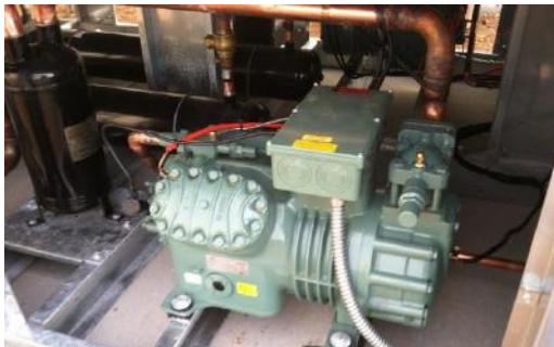
VFD driven Bitzer compressor
