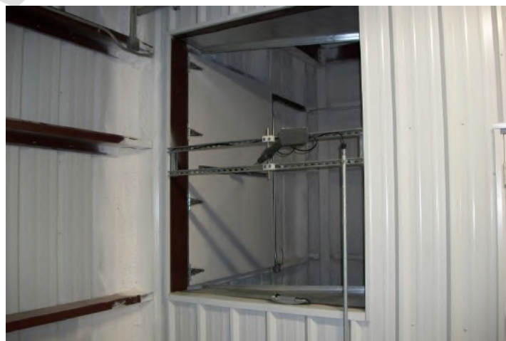
Intake fresh air door (inside view)
