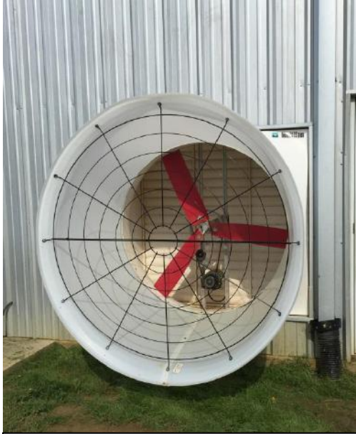
54" exhaust fan 30,000 CFM 1.5hp
