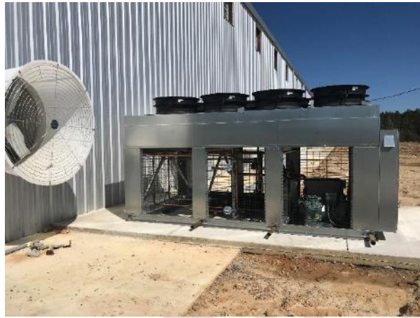
condensing unit with new style condensing fans
