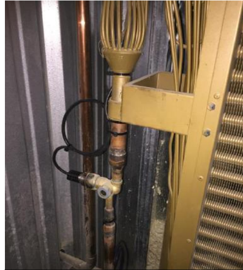
Electronic expansion valve
