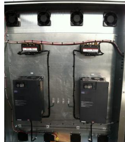
VFD's with TCI line filters
