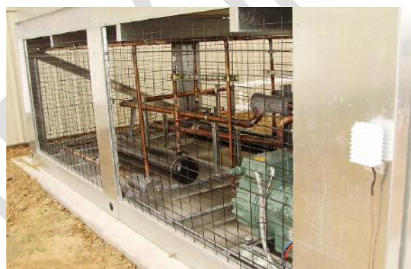
RSI refrigeration unit with Bitzer compressor
