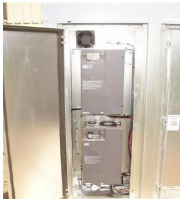
Refrigeration VFD's
