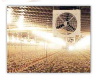
Notes: Fan can be mounted at any angle, this is an air circulator only.
